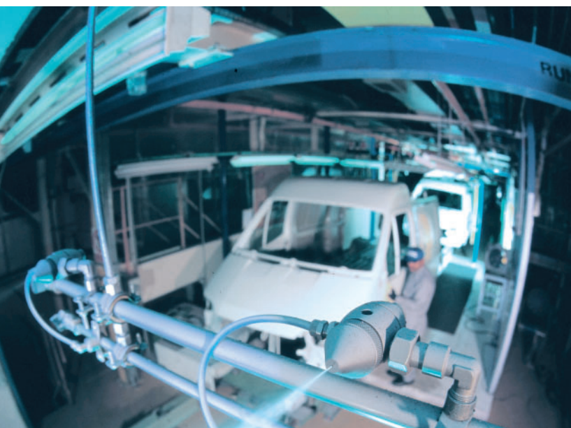
Humidification in an automotive painting plant
